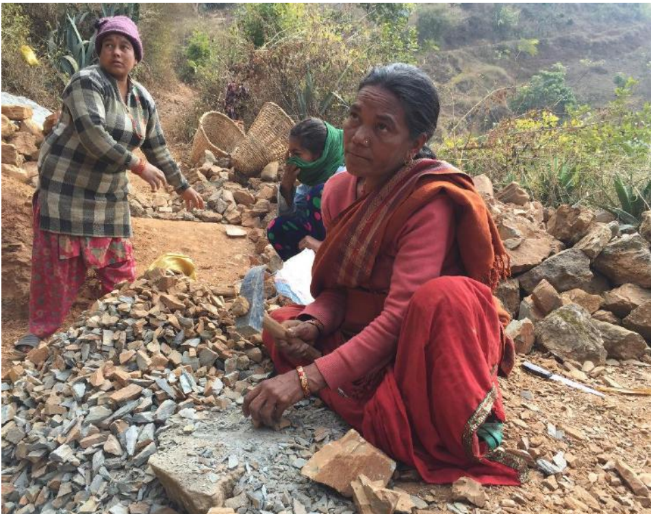
Women in Panchkhal, Kabhre, working on the reconstruction of the water supply system damaged by the 2015 earthquake. Photo: Ashim Poudel/KIRDARC.
